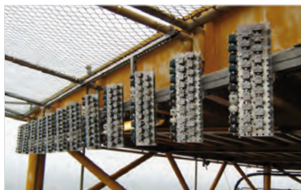
Field test in the Dutch sector of the North Sea
